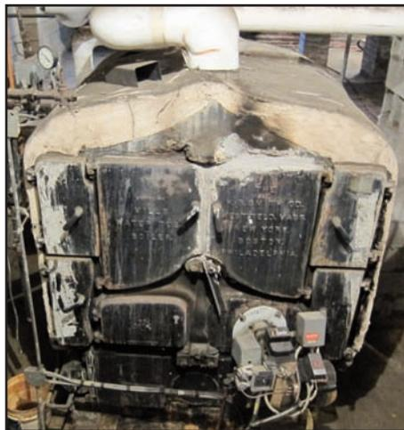
Well, we got a hundred years out of it. Not bad. The one million btu unit, pictured here, that has heated our sanctuary since 1911, finally developed multiple leaks this summer that couldn't be repaired. We will replace it with a one million btu gas fired unit.
